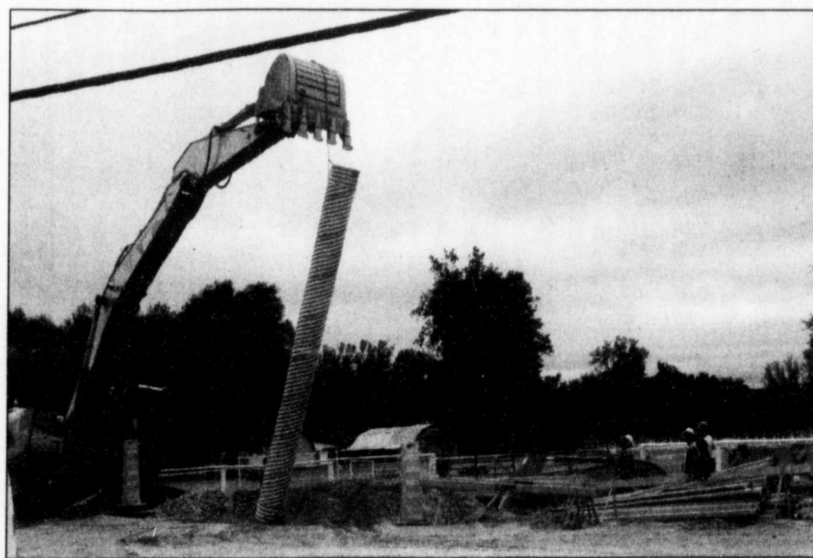
NEW AGE SEWAGE: Quyon's new sewer system is being installed here on Friday, July 23 at the intersection of Clarendon and Onslow Roads. The new system will include a lagoon filtration system that will stop any more sewage from being dumped into the
