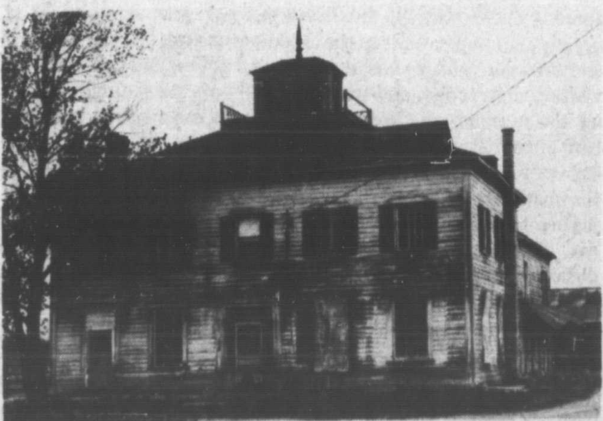
This historic wooden structure was once the home of Brysons in Fort Coulonge. The roof balcony was used by the ladies to watch up the Coulonge River and see where the men were, on their lumber drive towards the Ottawa. Quebec Cultural Affairs officials showed little interest in the restoration of this building, as they viewed it last Thursday. EQUITY PHOTO
