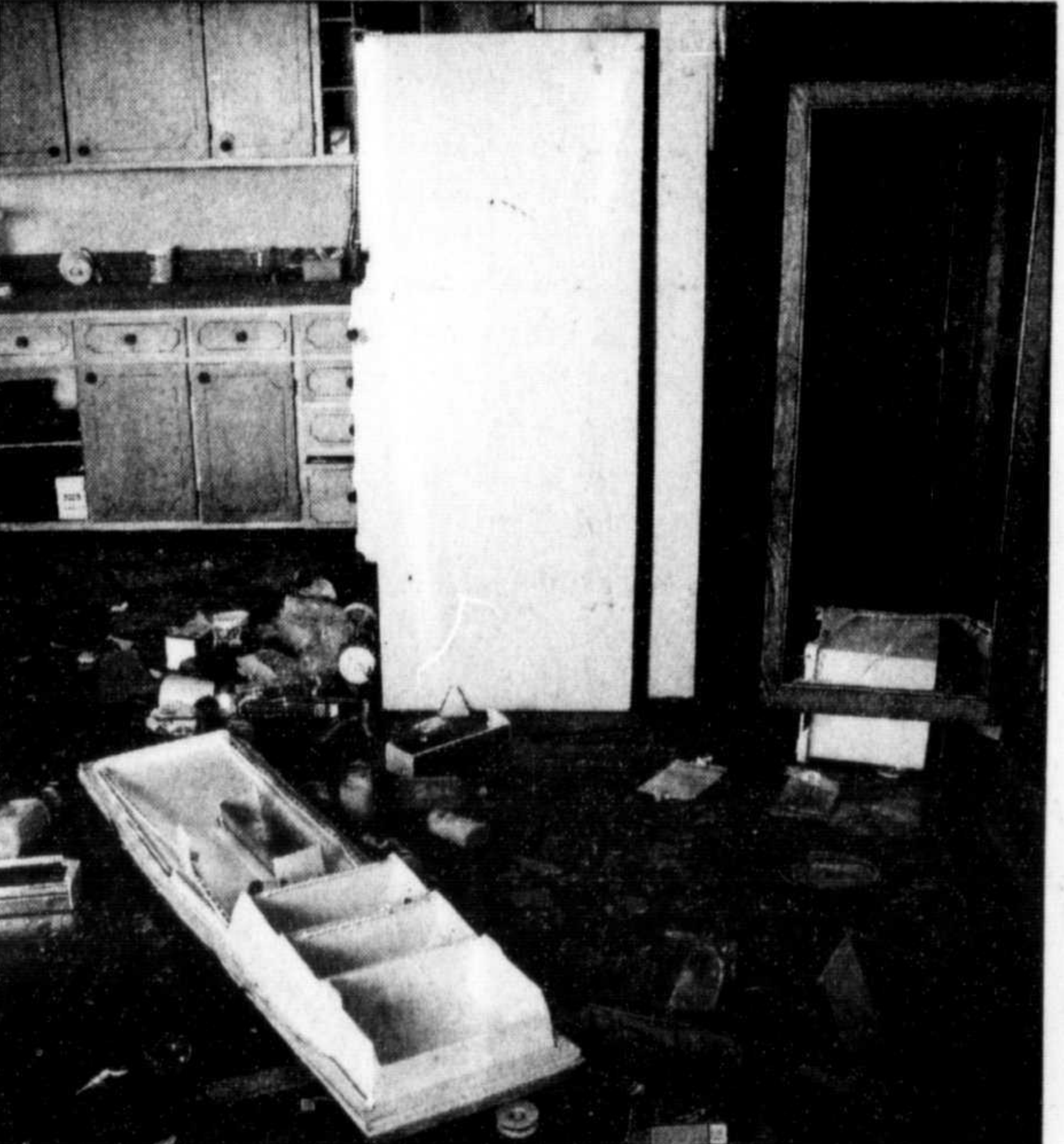
The damage to a cottage in Luskville caused a total of $20,000 worth of damage.
