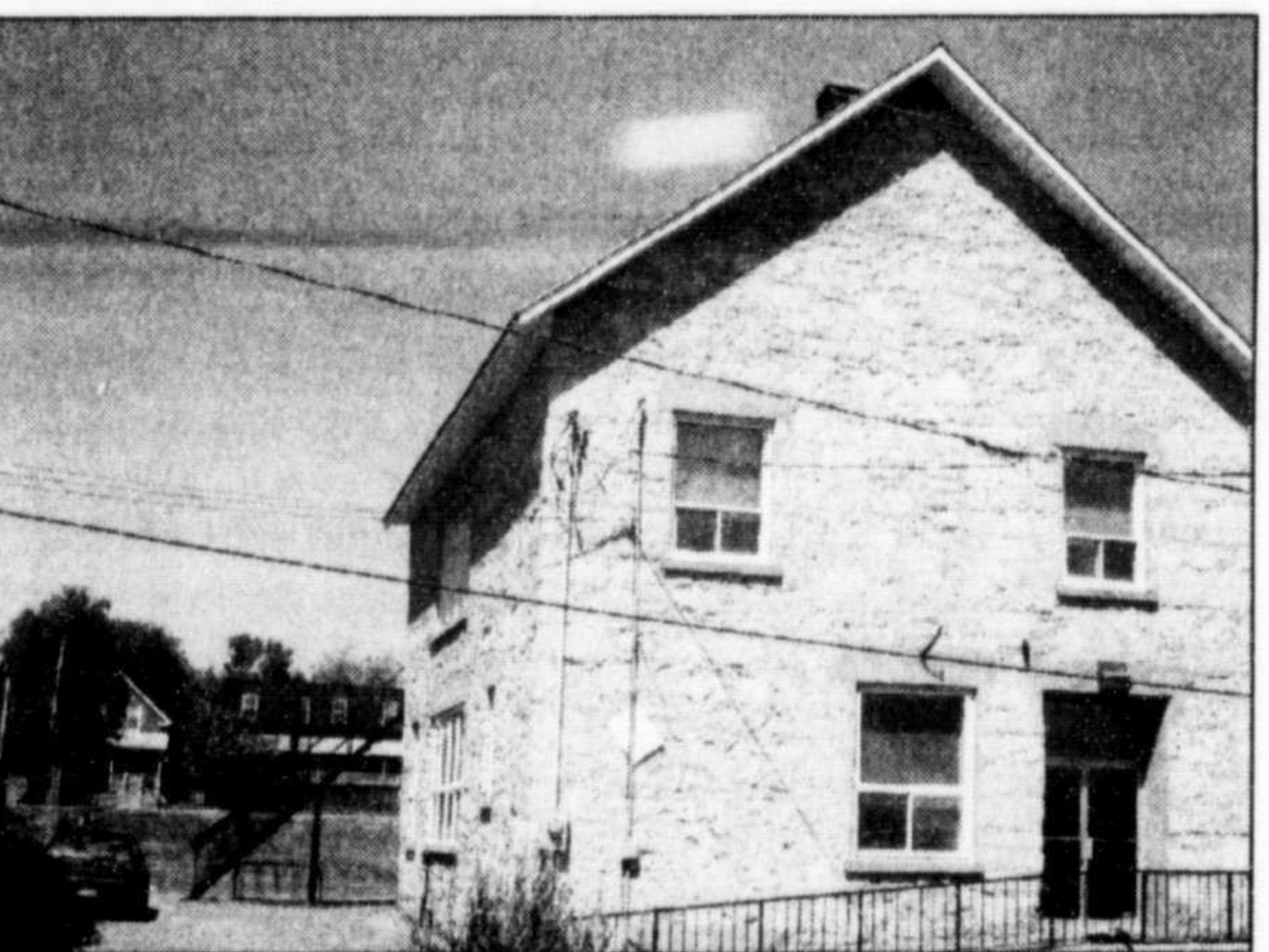
ABANDONED BUILDING: This old and abandoned building in Portage du Fort on Mill Street is ready to sell. After six months the building may be demolished.
