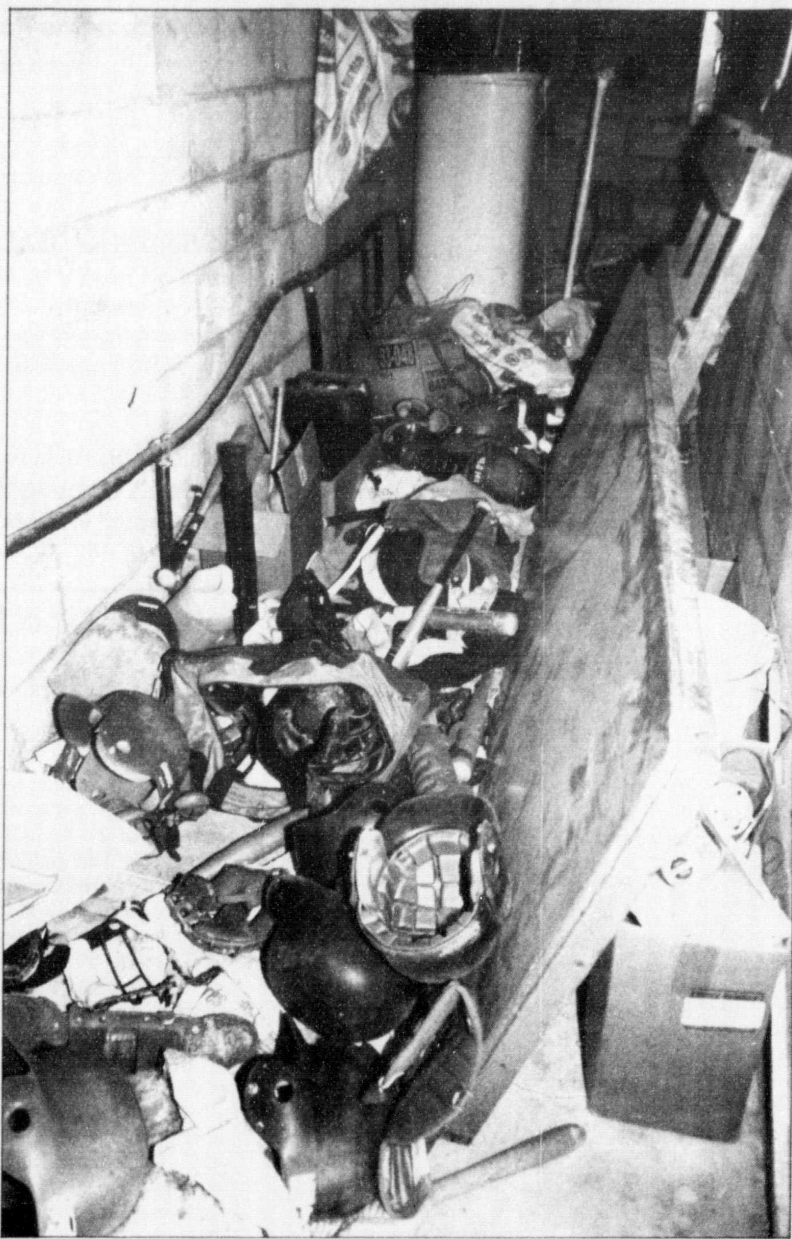
MINDLESS DESTRUCTION: The continuous mess and destruction left by vandals has forced the RA to tear down the building which holds the canteen and equipment room.
