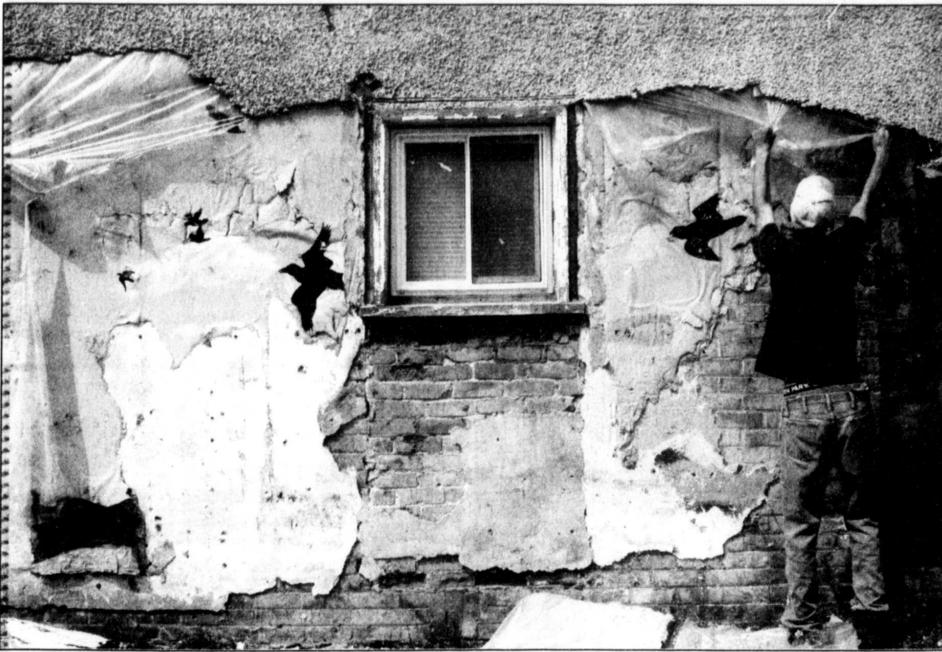
A renovator pulls down plastic that is covering an old mural that was found underneath the stucco of a house on Main Street.
