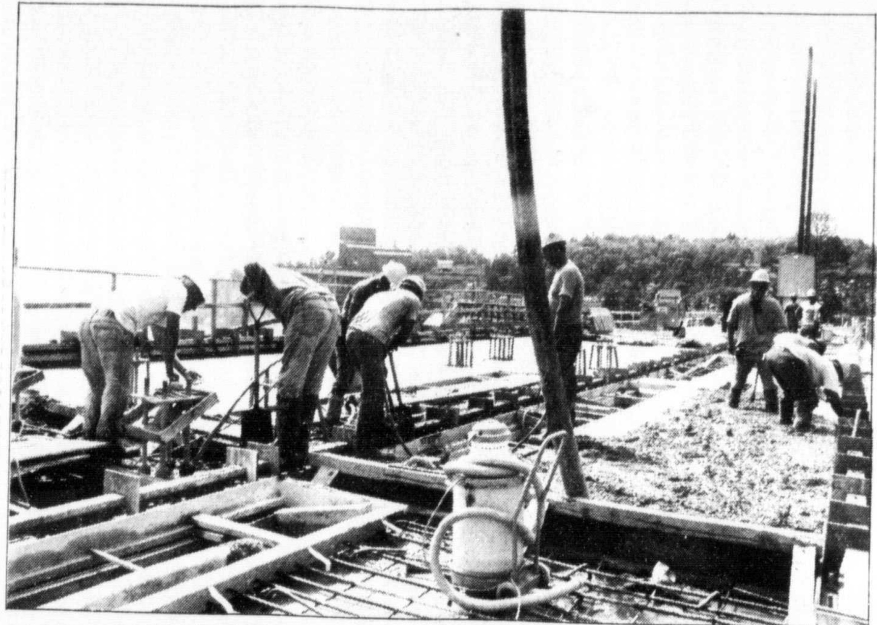
BRYSON DAM REPAIRS: Campbell's Bay Cement provided over 300 cubic metres of cement to the reconstruction of the Bryson Dam. The main cement pouring took place on Thursday, August 17 and due to the high temperatures ice had to be added to the cement to keep its temperature below 25 degrees Celsius.
