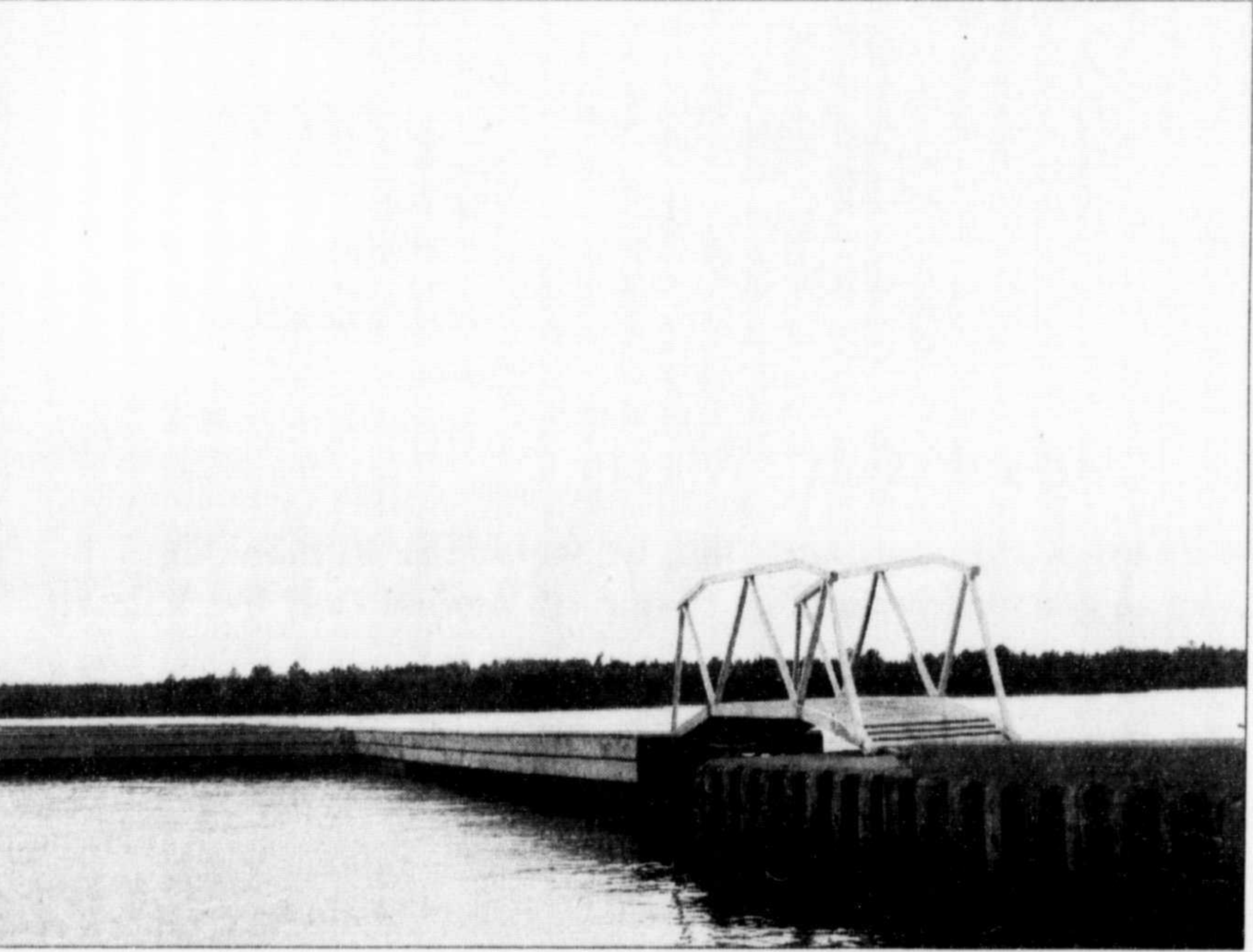
This new dock that was installed at Davidson is one of seven docks planned to be built this season.
